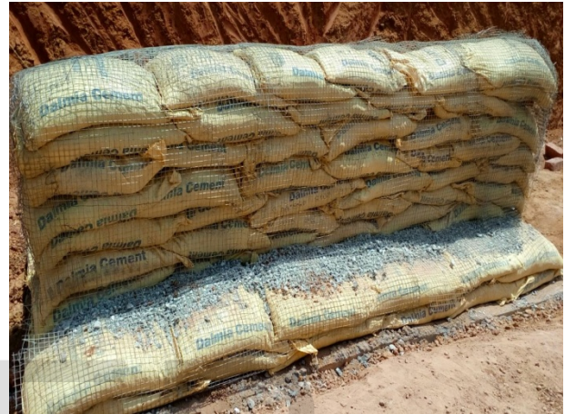
Fig: 3: Model of chicken mesh retaining wall (during construction)
